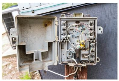
Figure 11-6 A Telephone System Demarcation Point
