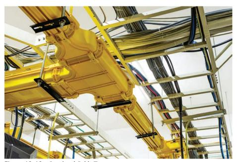
Figure 10-10 Overhead Cable Tray
